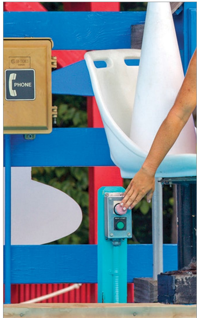
Figure 4-14 | An emergency stop (E-stop) button can be pressed to turn off the waves in a wave pool when a rescue is required.
